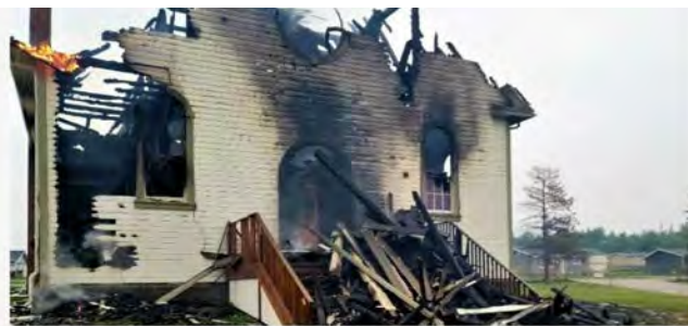
The loss of St. Bernard's Church in Grouard, Alta., makes a sad moment for those with memories of the church, said Grouard-McLennan Archbishop Gerard Pettipas. Two men have been arrested in connection with the fire. (Archdiocese of Grouard-McLennan photos)
